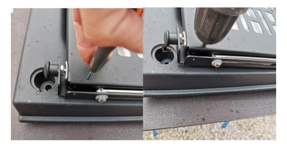
Drill hole in marked position using 5 mm drill bit.
